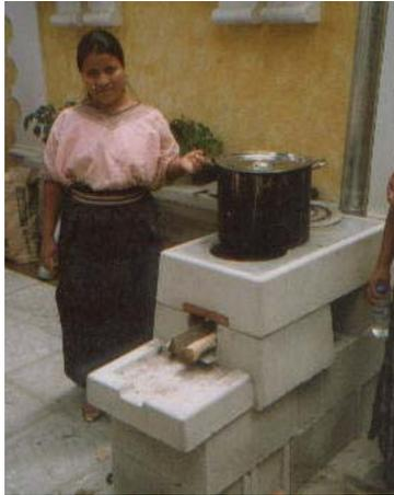
This cement Aprostove is being built by Helps International in the Guatemalan Highlands. Three individual cement pieces are cast in fiberglass molds and then assembled on site. The molds are easy to transport and help prevent design inconsistencies.
